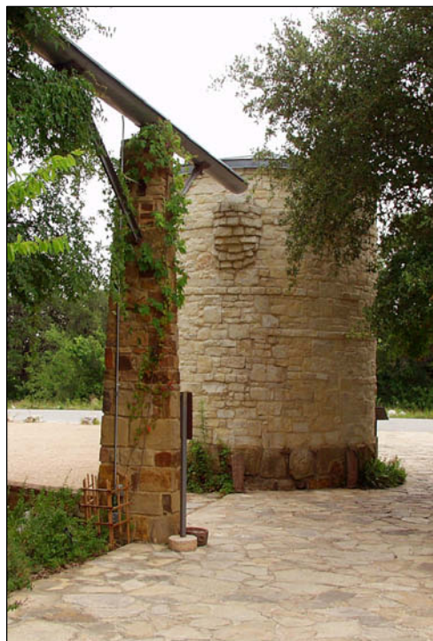
The entry cistern at the Lady Bird Johnson Wildflower Research Center is reminiscent of the stone-and-mortar cisterns used by Hill Country settlers. Water from a 1,200-square-foot roof area is conveyed to the entry cistern via an aqueduct.
